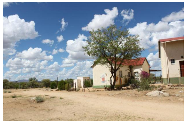
BEC site adjacent to the Church
